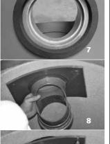
Insert, respectively hold the Funke-ILA (against the chamber wall) **(8)**, mark bore holes in the pre-tapped holes and create Ø 10 mm drills. Drill with stop, maximum 60 mm in deep - depending on the concrete chamber quality/wall thickness. Insert the supplied dowels and screw down the Funke-ILA in the intended positions **(9)**. If required install more dowels.
